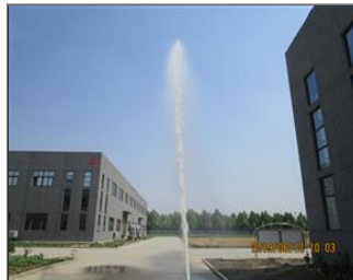
Photo of fire safety equipment Fire hydrant testing.JPG
