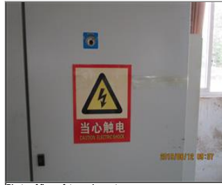
Photo of fire safety equipment Switch box with warning sign.JPG
